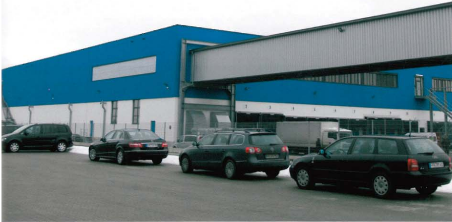
The production site of Glockenbrot in Bergkirchen has a size of almost 30,000 square meters.
