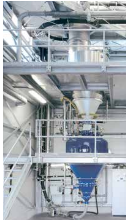
Discharge of powder from a pressure vessel.
